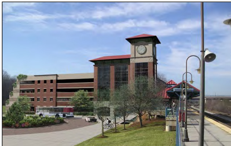
Burke Virginia Railway Express (VRE) Station.
