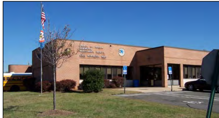
Picture of existing Newington facility
