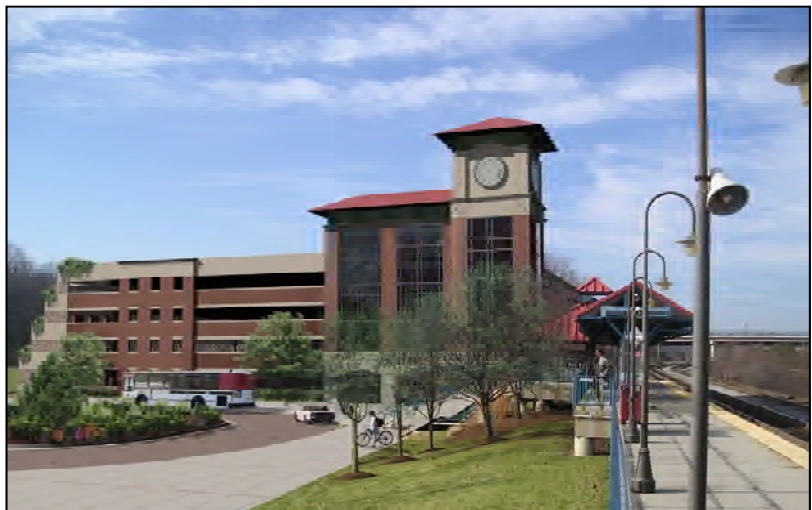
Burke Virginia Railway Express (VRE) Station.
