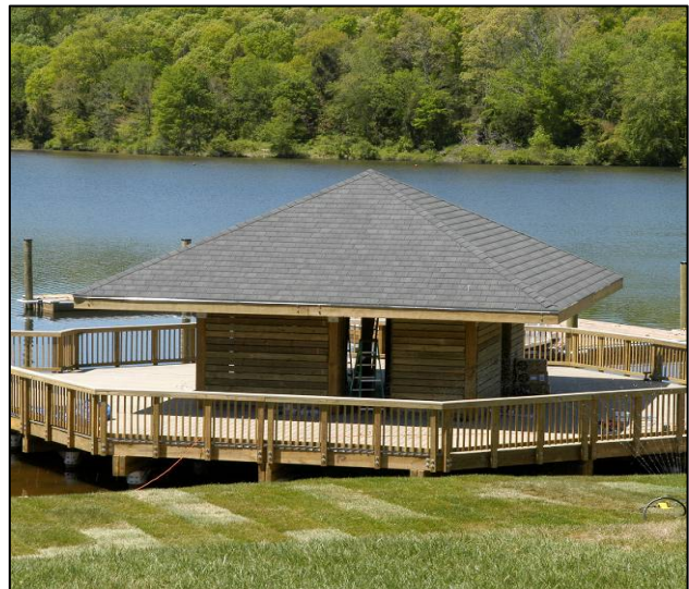
Picture of new dock at Lake Fairfax
