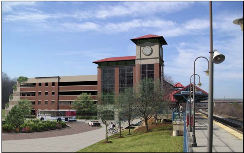
Burke Virginia Railway Express (VRE) Station.
