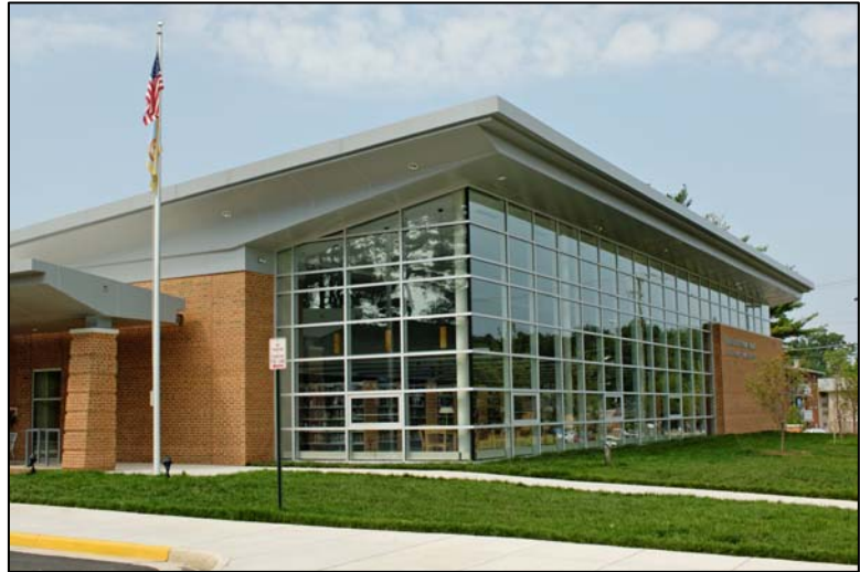
The renovation of the Thomas Jefferson Community Library, located in Falls Church, was completed in 2010. Photo credit: Paul Thornily.
