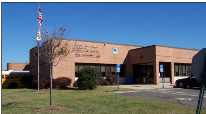
Picture of existing Newington facility
