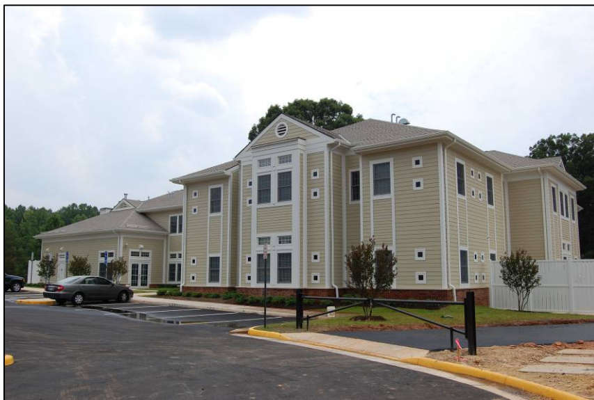
The new Katherine K. Hanley Family Shelter in western Fairfax County accommodates up to 20 families at a time.
