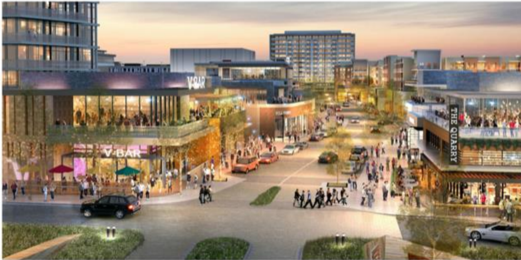
A rendering of the future entrance to Indigo Ridge North's Village District.
