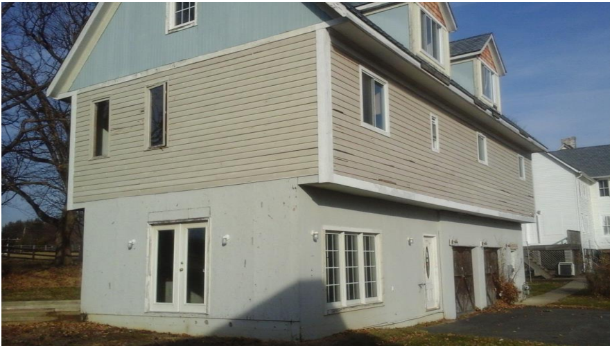
Caretaker's apartment and garage
