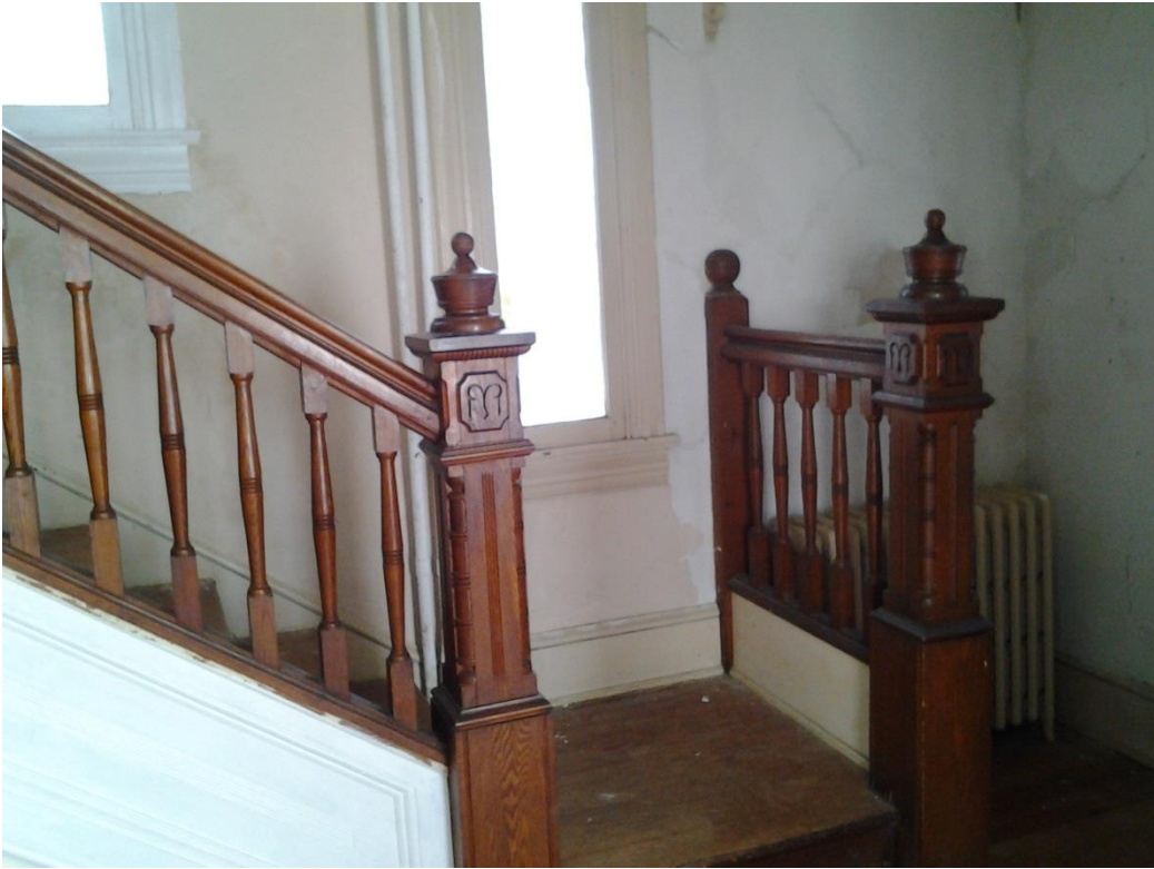
Turner Farmhouse Newel Post and Balustrade
