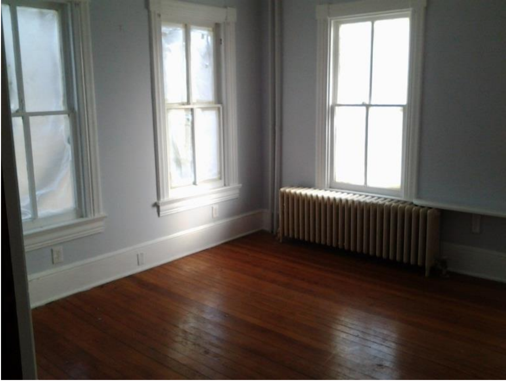
Turner Farmhouse First Floor Room 2
