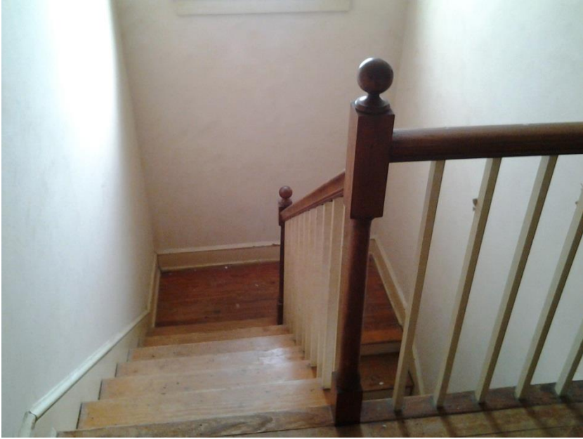
Turner Farmhouse "Servants Stairs"
