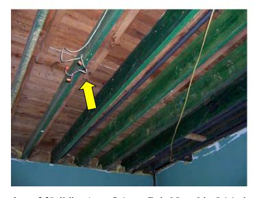
Image 2.29: Yellow Arrow Points to End of One of the Original Joists
