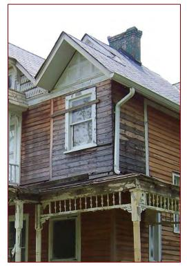
Image 2.12: Section of House Originally a Recessed Covered Porch
