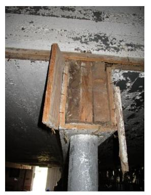
Figure 93. Ends of built up interior beam appear to be in good condition.
