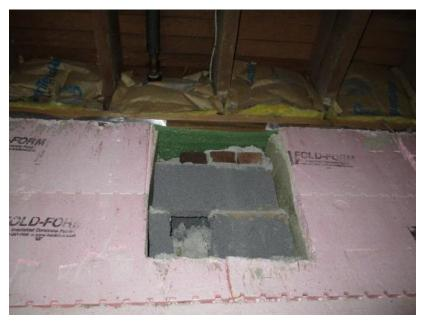
Figure 14. Blockout in cellar wall infilled with CMU, brick masonry, and grout.
