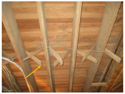
Figure 22. Disengaged and missing wood bridging between first floor joists (typical at original first floor framing).
