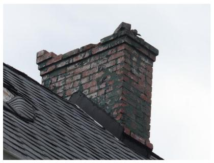
Figure 35. Missing and loose bricks at the chimney.
