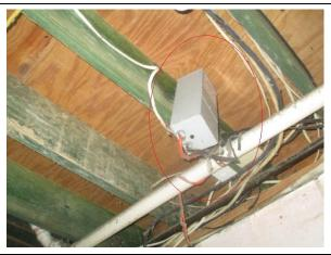
Photo 2: Abandoned box and wires in basement
