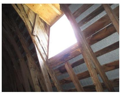
Figure 94. Deterioration of the wood framing at the central dormer along the west elevation.
