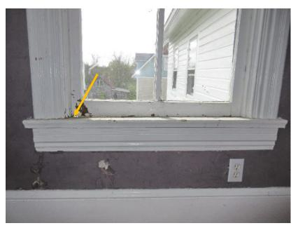
Figure 11. Typical staining and cracking below original window. Note this window is racked with visible daylight below the sash.
