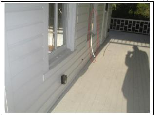
Photo 1: Loose cable near front door
