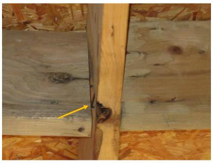
Figure 53. Gap is present between end of wood bridging and joist.
