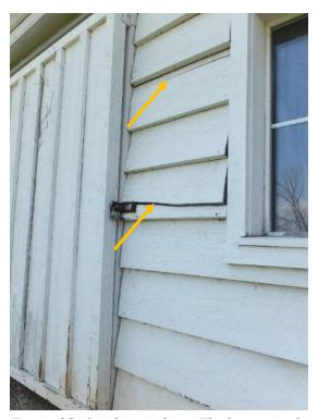
Figure 85. Cracks in siding. The lower crack is due to the installed latch.
