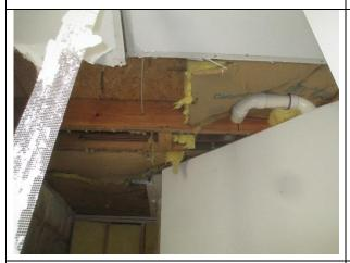
Photo 31: Water damage at mid-level ceilings due to water from floor above
