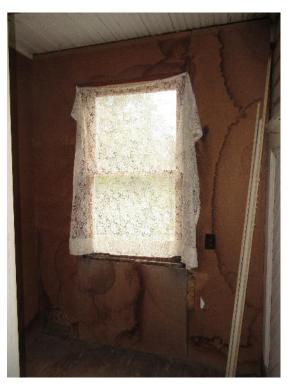
Figure 40. Deteriorated and stained particle board at the enclosed patio on the second floor.
