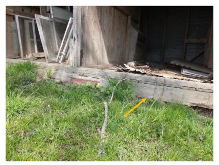
Figure 59. Timber sill bears directly on the ground.
