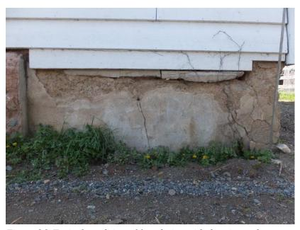
Figure 86. Typical condition of foundation with deteriorated parge coat and concrete spalls.
