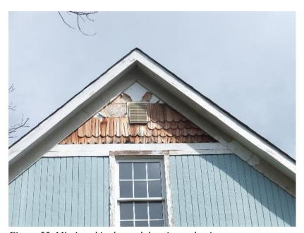
Figure 55. Missing shingles and deteriorated paint.
