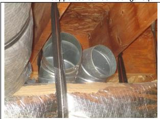
Photo 27: Duct fittings without dampers/diffusers
