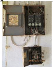
Photo 40: Derelict fuse box and wiring
