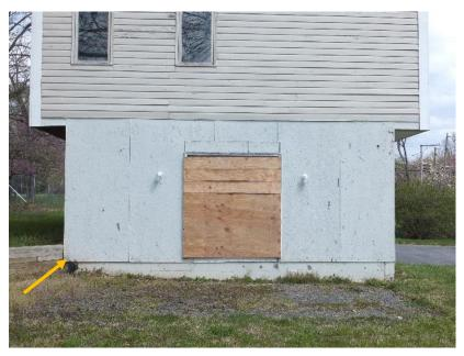
Figure 57. Exterior wood sheathing used for the southern addition to the garage.
