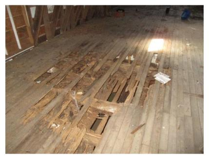
Figure 95. Deterioration of the wood floor boards below the central dormer along the west elevation.
