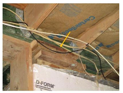
Figure 17. Built up wood blocking.
