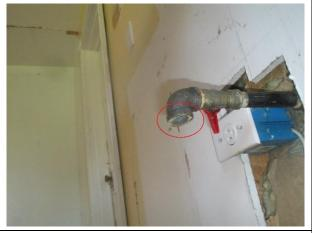
Photo 7: Kitchen gas piping through floor
