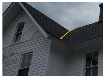
Figure 36. Asphalt shingles out of plane above the gutter.
