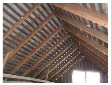
Figure 74. Roof framing as viewed from the loft.
