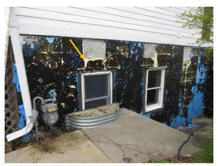
Figure 6. Deteriorated WRB and exposed insulation form where WRB is no longer in place.
