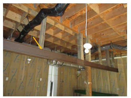
Figure 50. Steel beam runs longitudinally through the first floor of the north portion of the garage.
