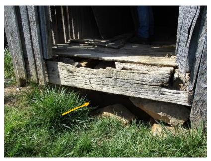
Figure 66. Large gaps are present in the stone foundation.
