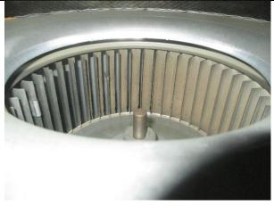
Photo 34: Condition of fan wheel at upper level heat pump unit
