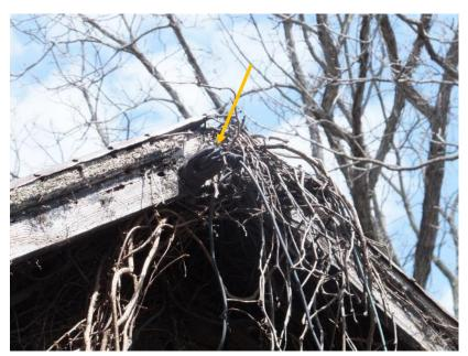
Figure 83. Lightning protection cable extended from the roof. Note heavy vegetation and damage to the fascia board.
