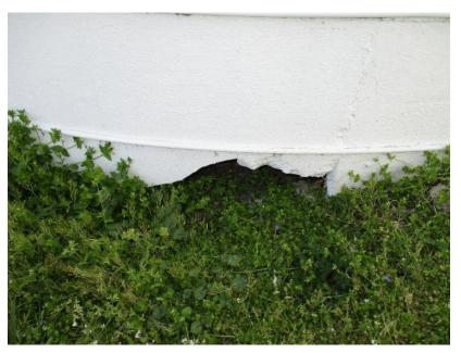
Figure 107. Concrete spall at the base of silo.
