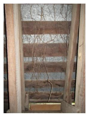
Figure 98. Vegetation between the roof framing and the metal roof.
