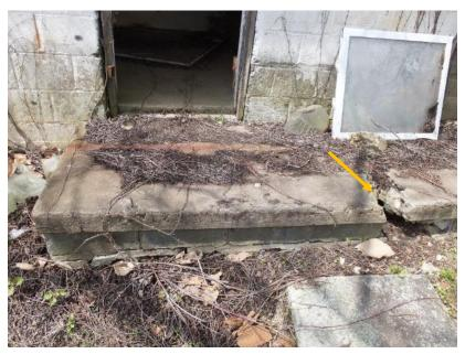
Figure 82. Large crack through concrete landing and deterioration of the supporting CMU.
