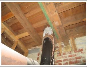
Photo 14: Flue thimble through floor above
