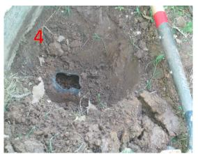
4. Garage sewer line is shown immediately outside west wall of garage. A small existing hole in the top of the pipe was enlarged to allow camera entry because the camera could not be pushed through the cast iron elbow inside the house. The camera could not be pushed more than 18" into the pipe at this location due to corrosion and debris. Recommend replacement of pipe to septic tank.
