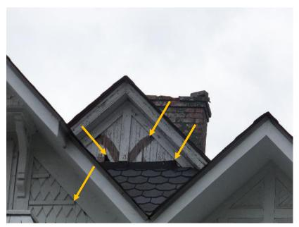
Figure 5. Roof felt at the secondary gable and roof shingles. Note hole in wood and profile from previous decorative trusses as well as miscellaneous horizontal wood boards on forefront gable.
