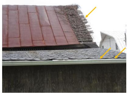
Figure 65. Missing metal roof section along with evidence of heavy vegetation. Note sagging asphalt shingles between rafters on the wing addition.
