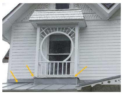
Figure 37. Lifted and separated flashing at Juliet balcony. Note gap between second floor flashing and porch roof.
