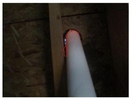
Figure 31. Daylight visible in attic around plumbing vent. Photo courtesy of MBP.
