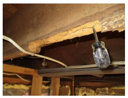
Figure 24. Deterioration at first floor joist in original farmhouse.
