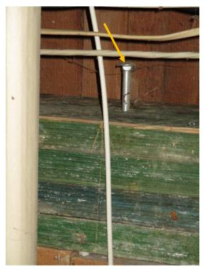
Figure 21. Disengaged bolt in built-up member.
