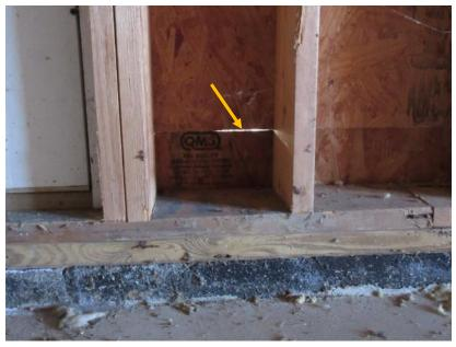
Figure 51. Daylight is visible between exterior wall sheathing panels in south portion of the first level.
