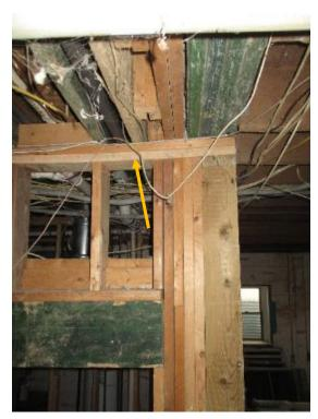
Figure 16. Deflection of header at interior partition wall.
