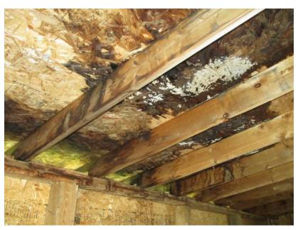
Figure 77. Staining, rot, and biological growth are visible on the underside of the plywood roof sheathing on the west lean-to addition.
