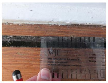
Figure 41. Split in flooring at the south wall of Room 102.
