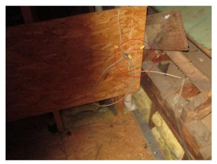
Figure 29. Unsecured wires in the attic. Photo courtesy of MBP.
