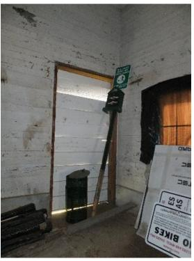
Figure 103. Evidence of previous door at the southwest corner of the barn. This would have connected to the silo.
