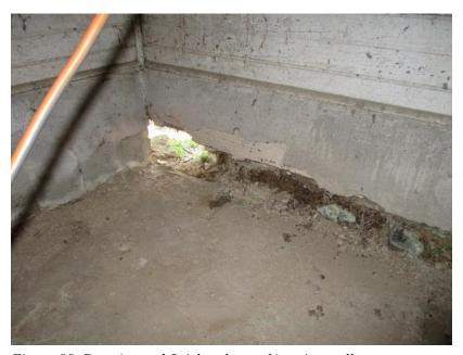
Figure 89. Deteriorated finish at base of interior walls.
