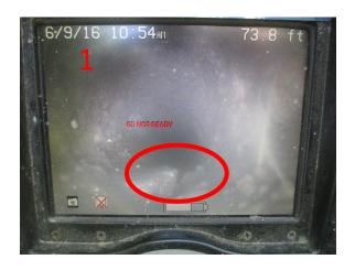
1. Septic pipe between tank and distribution box is broken at 74 feet, immediately west of sidewalk outside existing chain link fence.
