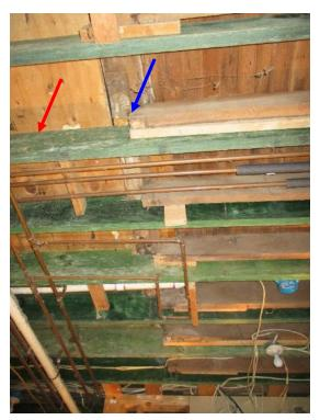
Figure 18. New framing members span the entire width of the south addition (red arrow). Original framing is no longer supported at west ends (blue arrow).
