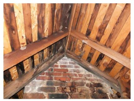
Figure 28. Staining in original roof wood framing adjacent to the chimney. Note the two types of brick indicating that the chimney may have been extended at one point.
