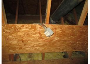
Photo 3: Unsecured wires in attic
