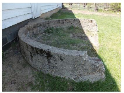
Figure 101. Concrete structure along east elevation of dairy barn. Note exposed reinforcing and concrete spalls.
