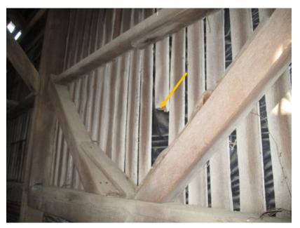
Figure 75. Fractured vertical wood slat.
