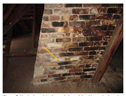
Figure 7. Vertical crack in the north face of the chimney in the attic.
