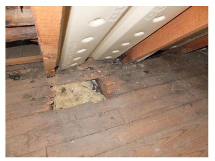
Figure 42. Deteriorated wood flooring in the attic.
