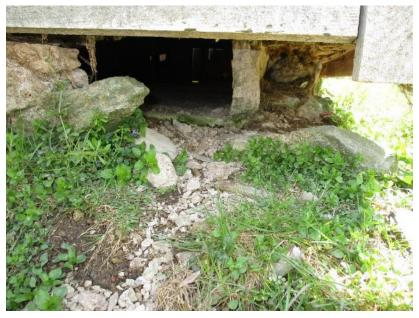
Figure 87. Stones present at foundation wall along west elevation.
