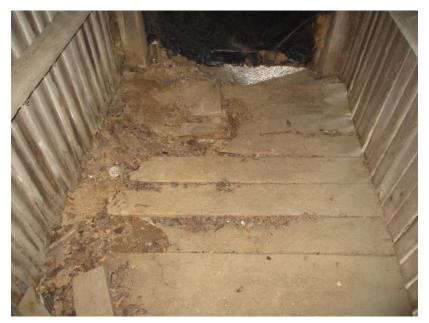
Figure 68. Floor joists and planks are in direct contact with the soil at the west crib.
