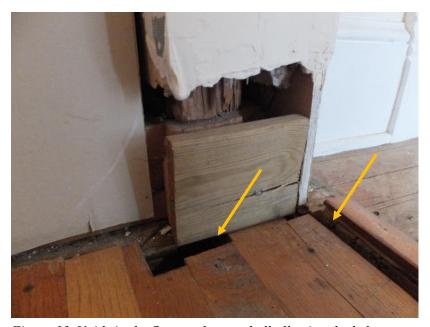
Figure 13. Voids in the floor at the rear hall allowing the below cellar to be visible. Note the missing baseboard and interior finishes at this location.
