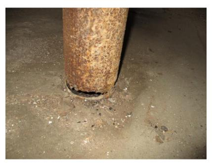
Figure 92. Section loss at base of pipe column.
