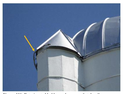
Figure 106. Deteriorated ladder enclosure roof at the silo.
