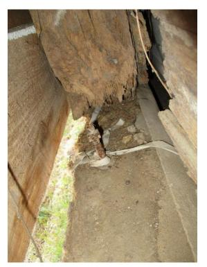
Figure 90. Loss of bearing at wood column.
