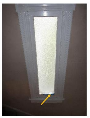
Figure 34. Broken glazing in stairwell fixed window.
