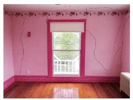
Figure 8. Example cracking in Room 201 at the north wall. Cracks have been traced for clarity.
