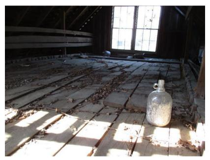
Figure 73. Rough sawn planks in loft.
