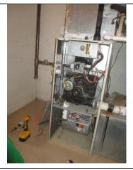
Photo 26: Condensate pump removed (lower left)
