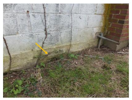
Figure 80. A small spall is present in the concrete foundation wall.
