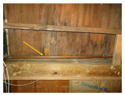
Figure 26. Staining and deterioration at first floor boards at the west edge of original farmhouse footprint
