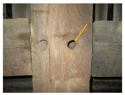
Figure 71. Missing wooden peg at interior connection.
