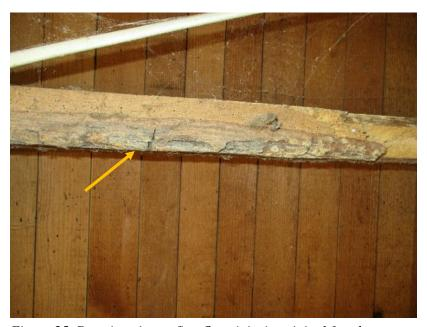
Figure 25. Deterioration at first floor joist in original farmhouse.
