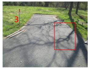
3. Existing parking space east of driveway should be removed. Septic distribution box is located in this area (shown approximate) and would be required to have a traffic rated structure if the parking area remains. Additionally, most local codes require separation between driveways and septic fields.
