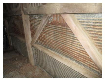
Figure 72. Surface corrosion present on corrugated sheet metal inside of east crib.
