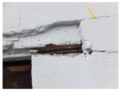
Figure 48. Corroded steel lintel and adjacent cracking in parge coat (orange arrow).
