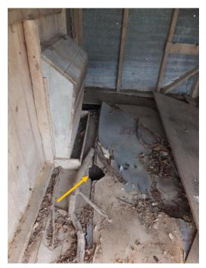
Figure 60. Complete section loss of the plank members along with the presence of an animal habitat, as evidenced by chew marks in a wood plank (orange arrow).
