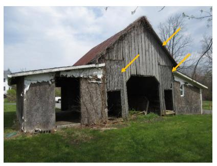
Figure 64. South elevation of the crib barn as viewed from the southwest. Note the historic wood slats and siding.
