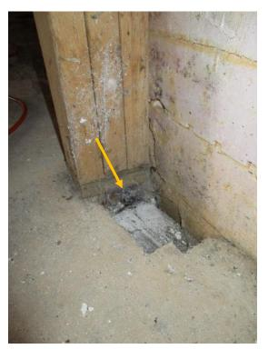
Figure 20. Void in concrete slab below column.
