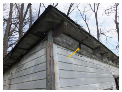
Figure 62. Rafter no longer bears on header.
