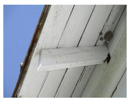
Figure 99. Deterioration at eave rafter.
