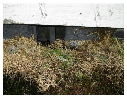
Figure 88. CMU present at foundation wall along west elevation.
