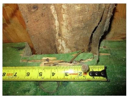
Figure 19. SCL joists are notched at their tops at what appears to be an old perimeter beam, which runs perpendicular to the joists.
