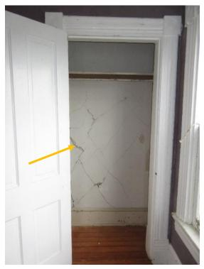
Figure 27. Diamond shaped cracking in closet of Bedroom 202.
