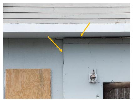
Figure 56. Gaps between the first and second floor and at the south addition.
