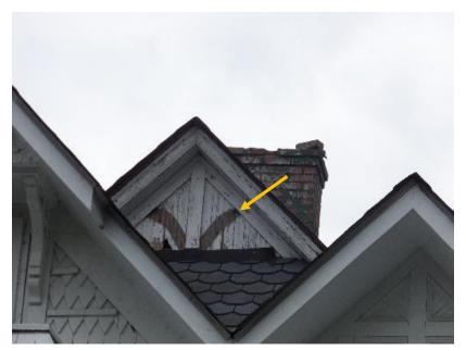
Figure 33. Deteriorated paint with evidence of previous decorative trusses at the secondary gable.
