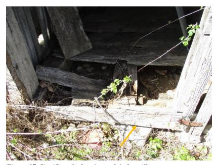
Figure 67. Significantly deteriorated timber sill.
