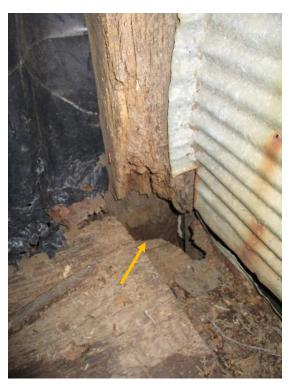
Figure 70. Nearly complete loss of bearing at the northeast corner column in the east crib.
