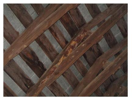
Figure 97. Isolated deterioration at truss framing member.
