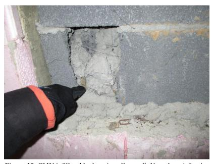
Figure 15. CMU infill at blockout in cellar wall. Note the reinforcing bar present inside the damaged cell.
