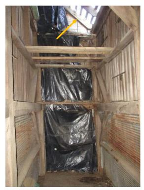
Figure 69. A portion of the metal roof is missing at the northeast and corner of the original structure.
