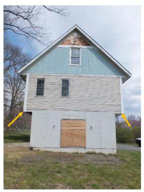
Figure 47. South elevation of garage. Note the overhang at the second floor line.
