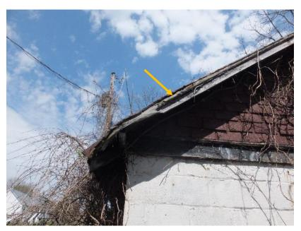
Figure 81. Exposed wood framing is in poor condition.
