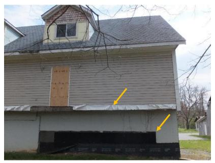
Figure 46. Exposed roof underlayment (black) and building paper (white).
