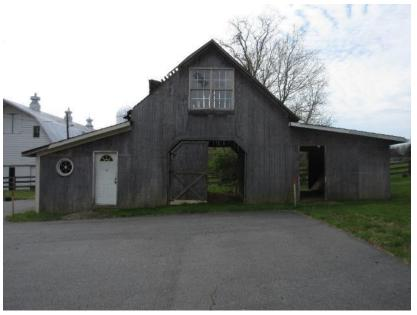
Figure 63. Crib barn as viewed from the north. Note the two "wings" adjacent to the central bay are not original to the structure.
