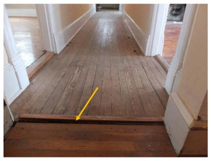
Figure 12. Transitions between Hallway (100) and adjacent rooms. Note gap between the rear hall to the Hallway (100).
