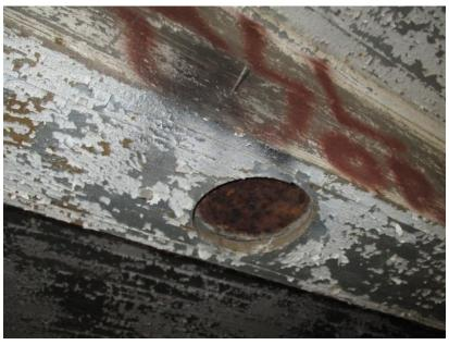
Figure 91. Missing pipe column.
