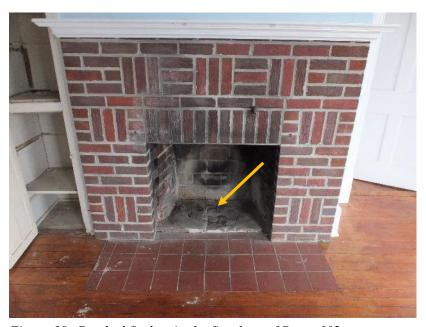
Figure 39. Cracked firebox in the fireplace of Room 102.
