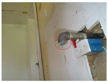
Figure 32. Gas piping improperly terminated in the kitchen. Photo courtesy of MBP.
