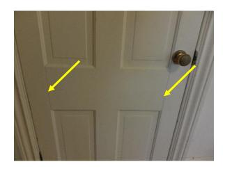
Figure 90. Separation of joinery at original door, typical.
