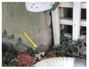
Figure 20. Spall in parge coat at original foundation exposing stone foundation.
