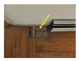
Figure 84. Exposed wood from pre-existing hallway structural elements. Note intersecting floors.
