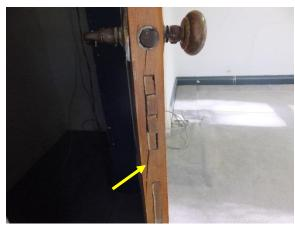
Figure 92. Splitting on stile of door facing latch, at D205.
