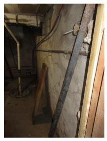
Figure 76. Northwest wall of cellar bowed out of plane and cracking in parge coat. Typical on northwest side of cellar.
