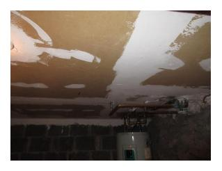
Figure 70. Drywall compound installation at gypsum ceiling panels in cellar.
