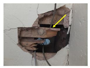
Figure 54. Hole through plaster and lathe for wiring.
