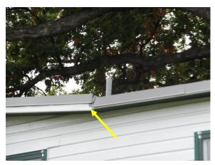
Figure 33. Displaced roof coping on southeast facade.
