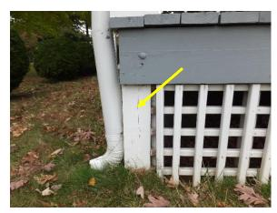
Figure 36. Vertical separation (checking) at wood porch column.
