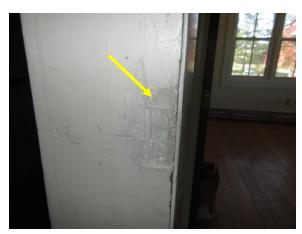
Figure 64 Tooling damage at wood siding panel at entry area adjacent to Room 209 & 210 (offices).
