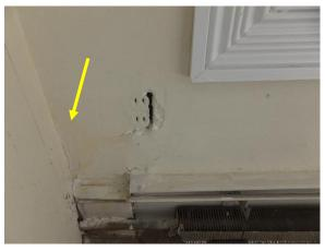
Figure 56. Stained plaster and potential previous repair. Note electrical outlet.
