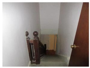
Figure 68. Drywall covering enclosing the historically open original stairwell and handrail.
