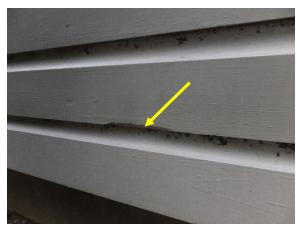
Figure 16. Chipped wood siding at base of siding at northeast facade.
