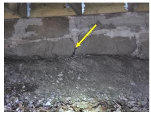
Figure 40. Missing mortar in stone foundation.
