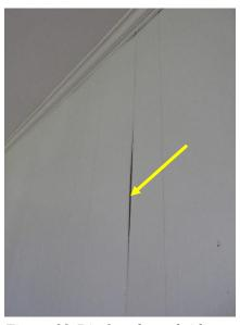
Figure 66. Displaced wood siding panel, typical.
