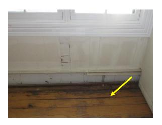
Figure 86. Staining at wood floor in Room 210 (office). Split across flooring visible.
