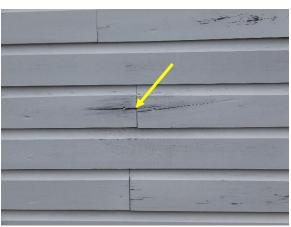
Figure 14. Typical cracking at fastener and end of boards.
