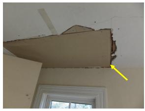
Figure 52. Removed area of plaster with drywall patch in room 201 (bedroom).
