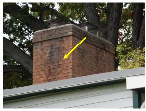
Figure 28. Staining at chimney located at the rear of the 1945 addition.
