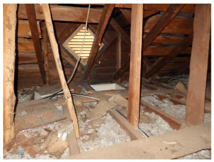
Figure 2. Framing of original attic access.
