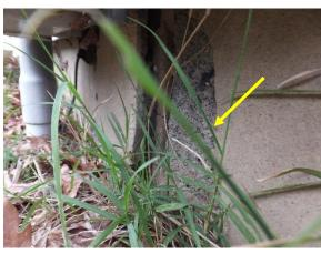
Figure 24. Delamination in parge coat exposing CMU foundation between ca. 1945 and 1984 additions on southeast facade.
