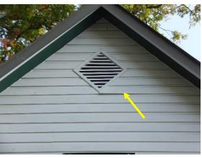
Figure 12. Example of displaced siding at southwest facade.
