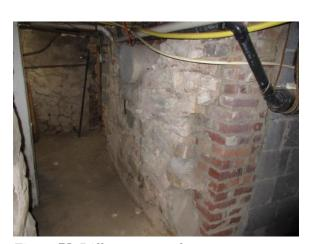
Figure 75. Different types of masonry construction in cellar fieldstone, brick, and CMU.
