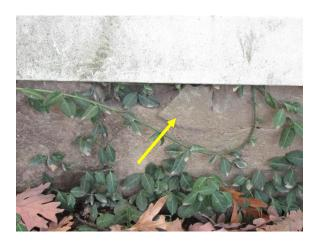
Figure 21. Incipient spall in parge coat at original foundation near window well.
