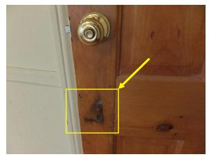
Figure 94. Missing original rimlock at D101
