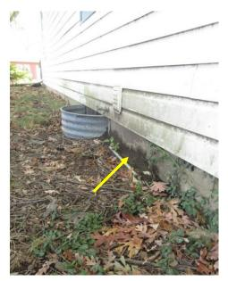
Figure 22. Foundation wall concave at original foundation. Note vegetative growth and staining at parge coat and above siding.
