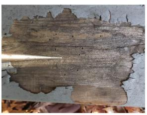
Figure 38. Paint and wood deterioration at porch stairs.
