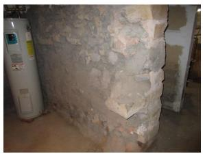
Figure 77. Deteriorated mortar and previous patch repairs at original stone foundation wall in cellar.
