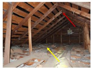
Figure 74. Rafter stud supports not continuous (yellow arrow) in attic and toe-nailed rafters (red arrow).
