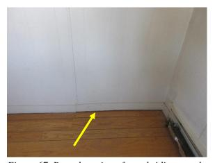
Figure 67. Bowed portion of wood siding panel in Room 210 (office).
