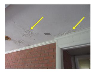
Figure 57. Damaged drywall due to water infiltration
