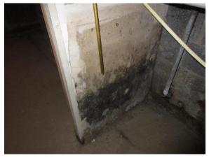
Figure 71. Potential microbial growth at drywall in cellar.
