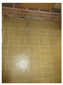
Figure 89. Delaminated and damaged linoleum flooring, typical.
