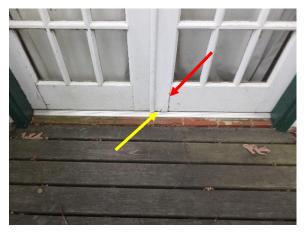
Figure 29. Splintered wood at base (yellow arrow) and separation of joinery (red arrow) at French doors.
