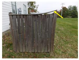
Figure 42. Bowed top rail of fence at southeast facade.
