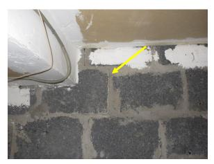
Figure 79. Bondline failure at CMU foundation wall in cellar.
