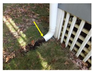
Figure 34. Downspouts terminate near the foundation without splash pads or extensions and have eroded the adjacent soil, typical.
