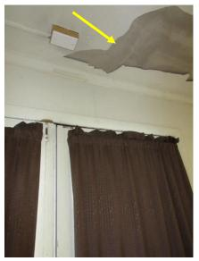
Figure 58. Drywall delamination at rear entryway.
