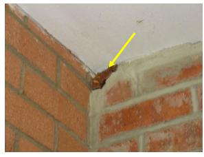
Figure 82. Spalled brick infilled with wood piece at Room 107 (bedroom).
