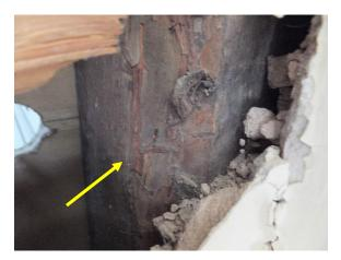
Figure 55. Original timber framing.
