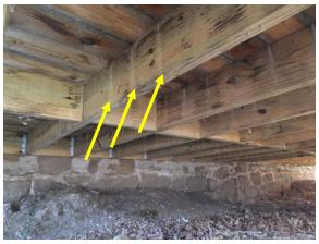
Figure 39. Wood joists under porch exhibiting staining, likely from water.
