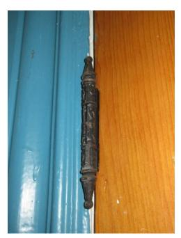
Figure 95. Original ornate steeple door hinge at D207.
