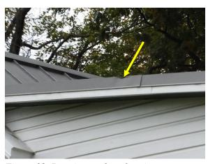
Figure 32. Dent in metal roof coping on southeast facade.
