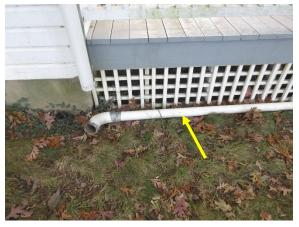
Figure 35. Disconnected downspout at northwest facade.
