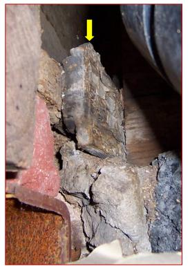
Image 3.65: Exterior Siding Observed Where the Joists for the Rear Stairs Attach to the Back of the House at the Kitchen
