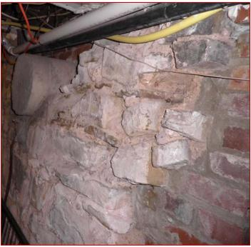
Image 3.18: Original Foundation Cellar Wall That Has Been Modified
