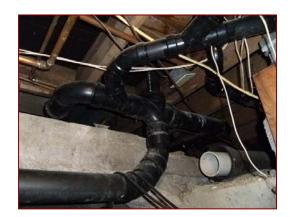
Image 4.17: Sanitary Sewer Piping
