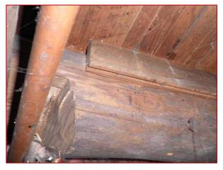
Image 3.2: Yellow Pine Log First-Floor Joists
