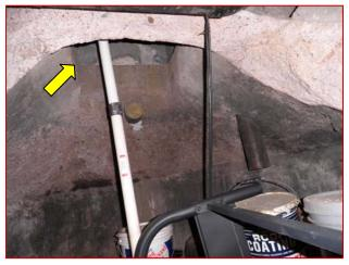
Image 3.74: Opening at Top of Septic Tank
