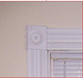
Image 3.69: Window Trim Cut on an Angle, Rather than Square, for Installation of Corner Block
