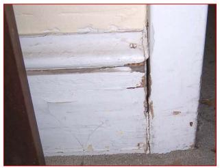
Image 3.83: Re-nailed Baseboard and Base Molding
