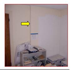
Image 3.68: Wall Extends Into Bedroom 202 to Increase Original Width of Hallway
