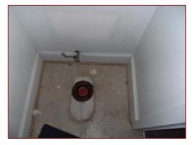
Image 4.20: Capped Sanitary Sewer Line
