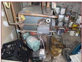
Image 4.11: Oil-fired Hydronic Boiler
