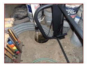
Image 4.19: Sump Pump Within Floor Drain
