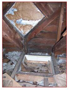
Image 3.73: Framing for Original Attic Access
