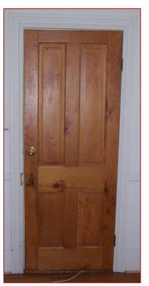
Image 3.4: Original Door D103, Similar to Other Original Doors A few of the original doors still have original door hardware. Other original doors had their locksets replaced with a knob handle and recessed-latch type hardware. Door D103 has an upright rim lock on the interior side of the bedroom door with a brass knob on the other side below a modern deadbolt.
