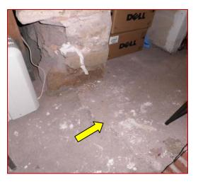
Image 3.60: Joint of Two Concrete Pours
