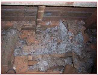
8. The original roof sheathing indicates that the roof was patched after the chimney was removed.
