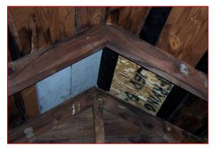
Image 3.63: Roof Patch at Earlier Chimney Location
