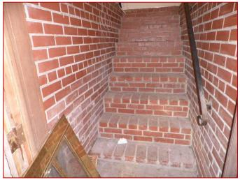
Image 3.19: Enclosed Brick Masonry Stair
