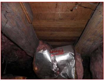
Image 3.21: Log Joists in Original Portion of House
