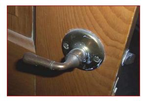
Image 3.8: Brass Lever Handle on Closet Door D206, Closet Side
