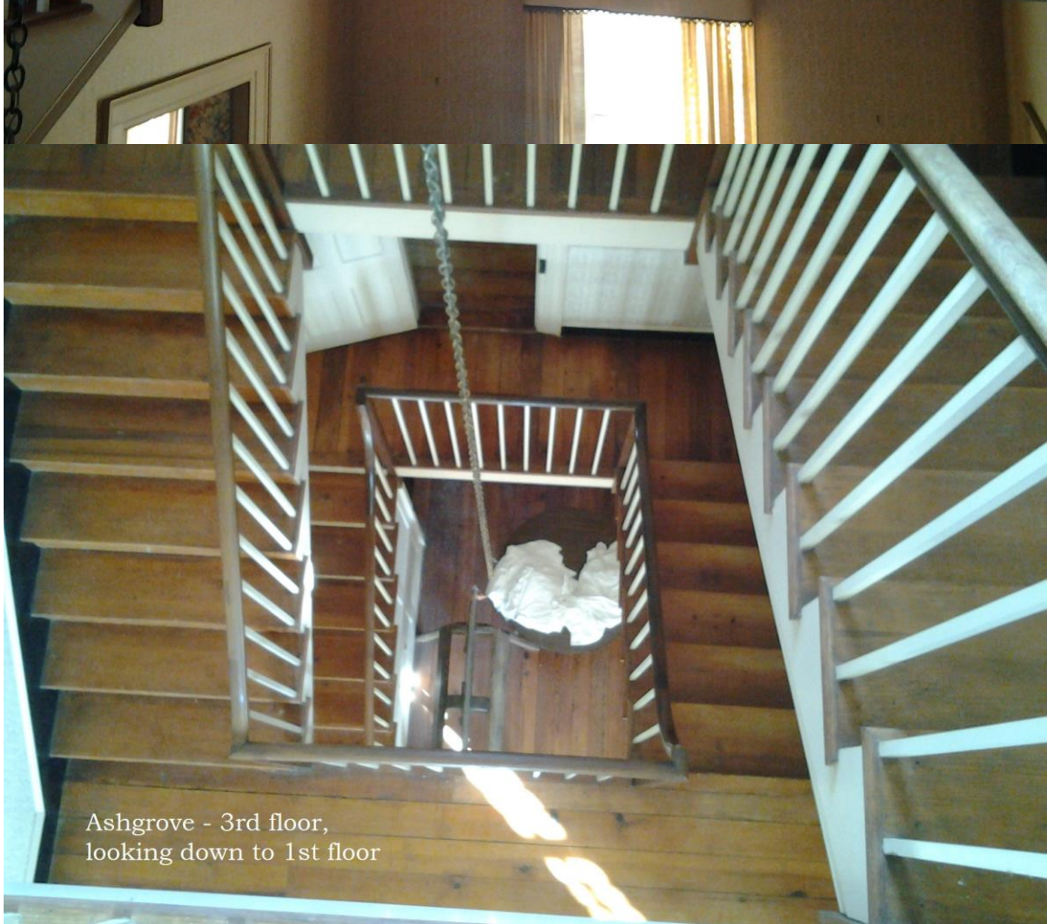
Ashgrove - 3rd floor landing view of duct work for HVAC system
