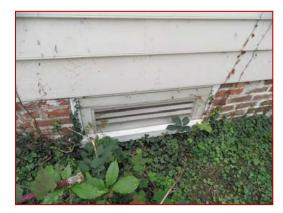
The crawl spaces are open to the basement and the original crawl space ventilation openings have been covered with plexiglass. The basement does have supply registers as described in the second HVAC system above.
