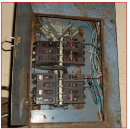
There are two 200A panelboards in the basement. The panelboard on the left feeds HVAC/Furnace loads (two pole loads) and is the newer panel, although neither is dated. The 200A panelboard on the right, which appears to have been installed as part of the 1960s renovation, feeds the kitchen and other building receptacle loads. Both panelboards have extensive exterior rust damage which implies the interior of the circuit breakers are also rusted. The panelboards should be replaced.
