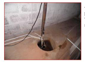
The condensate drain piping for the HVAC air handling units discharges into a pit with a sump pump. The sump pump appears to discharge to the sanitary system. The pit does not have a lid.
