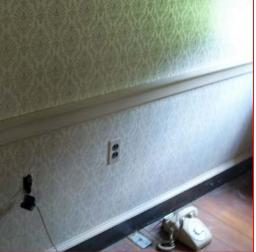
The NEC also requires one receptacle per 12 linear feet of wall space, which has not been strictly met in the building. Dedicated kitchen circuits are also now required by the NEC as well a minimum of two dedicated above-counter receptacles. The above counter receptacles are in place, but the circuiting was not verified.
