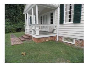
The roof has gutters with downspouts that discharge directly onto grade. There are no splash blocks.
