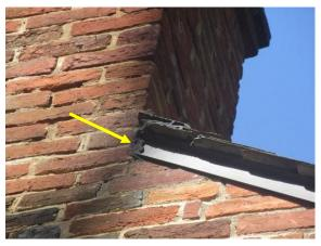
Figure 280. Mastic at south rake edge.
