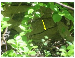
Figure 260. Crack in fieldstone.
