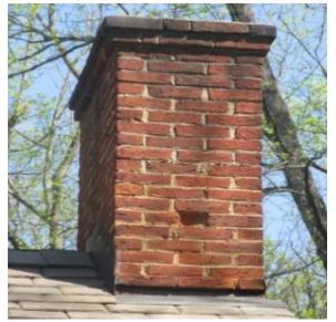
Figure 272. Erosion of brick face material.
