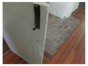
Figure 184. Slide bolt at the interior of north lower cabinet door.
