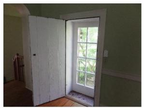
Figure 71. View of the exterior of the board and batten bead door in the Parlor with glass lite storm door.
