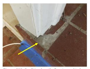
Figure 388. Spall in clay tile flooring at kitchen entry that has been covered with mortar.
