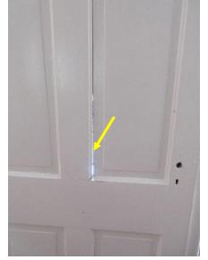
Figure 310. Daylight observed at exterior door panel.
