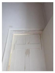
Figure 346. Flaked paint at interior door.
