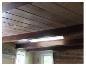
Figure 106. Exposed floor beams and subfloor in kitchen.
