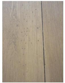
Figure 382. Potential insect damage at floor board in the living room.
