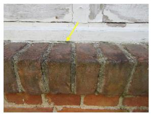
Figure 295. Deteriorated window perimeter sealant.
