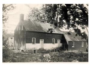
Figure 42. Historic photograph during abrasive removal of white wash during September 1948.
