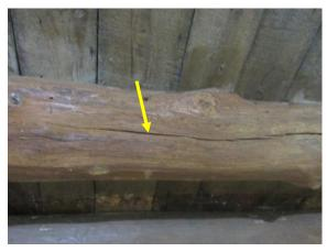
Figure 375. Checking at original floor beam in cellar.
