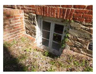
Figure 53. Typical cellar paired casement window.
