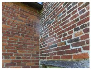
Figure 48. Interface between the original section of the home (right) and 1941 addition (left).
