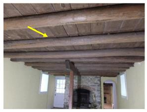
Figure 122. Exposed 3/4 round floor beams run north-to-south. Note shadowing adjacent to beams.
