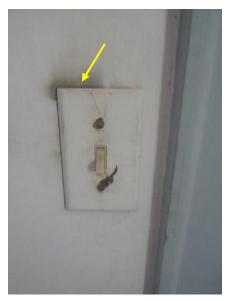
Figure 330. Black burn marks at electrical switch.
