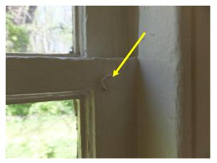
Figure 59. Sashes secured together at the interior.
