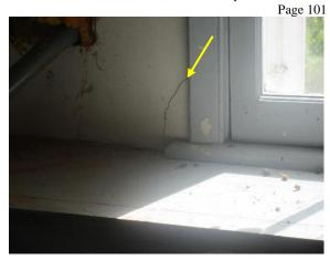
Figure 319. Plaster cracking adjacent to window frame.
