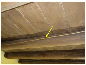
Figure 374. Splitting at 3/4 round wood floor beams.
