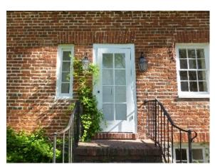
Figure 76. 4-paneled door at the south facade with glass lite storm door.
