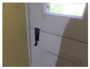
Figure 84. Typical interior door hatch at dutch doors.
