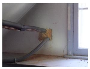
Figure 254. Mechanical conduit penetration through the east wall.
