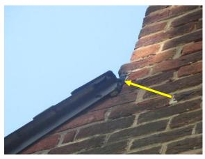
Figure 281. Mastic at north rake edge.
