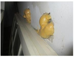
Figure 392. Abandoned penetrations at west loft bathroom infilled with spray foam.
