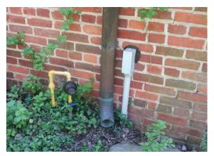
Figure 288. Downspout close to masonry wall.
