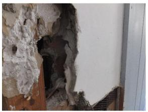
Figure 241. Plaster as observed at removed tub location.
