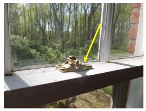
Figure 66. Brass sash locks present at 6/9 double hung windows.
