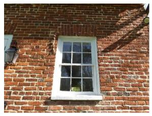
Figure 54. Typical 6/6 double hung window at the original section of the home.
