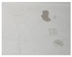
Figure 343. Typical cracked and flaked paint.
