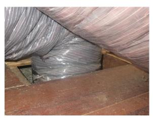
Figure 385. Cut in wood flooring to accommodate ductwork at east loft.
