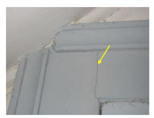
Figure 357. Separation of joinery at board and batten door frame.
