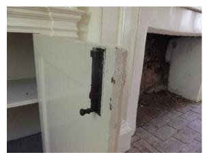
Figure 214. Slide bolt at interior side of south door.
