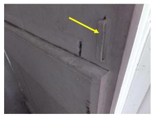
Figure 190. Interior side of stairwell door with strap for thumb latch lever remaining.
