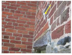
Figure 274. Step cracking was repaired with mortar at the ground floor/cellar door.
