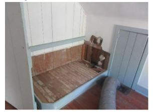
Figure 324. Cut in plaster and beaded wood wall for plumbing in west loft.
