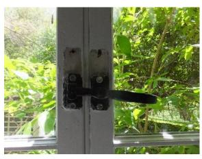
Figure 58. Casement latches at the ground floor windows.
