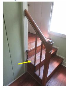
Figure 368. Missing spindle at parlor staircase.
