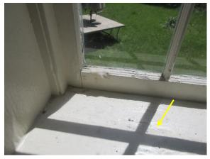
Figure 299. Weather-checking at window sill (interior).
