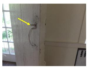
Figure 80. Thumb latch and handle remaining in Hall.
