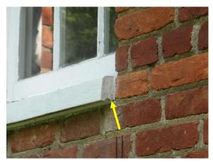
Figure 69. Wood sills at the addition with drip edges.
