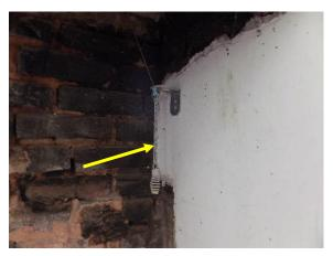
Figure 210. Typical damper pull chain.
