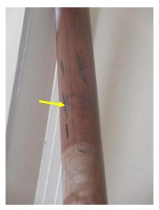
Figure 367. Indentations at a stair handrail in the hall.
