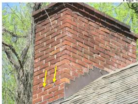
Figure 269. Sealant at mortar joint.
