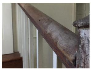
Figure 223. Profiled handrail along steps to loft stairs.
