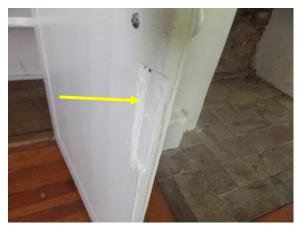
Figure 185. Removed hardware location below slide bolt.
