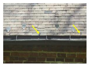
Figure 282. Mastic at slate joints.
