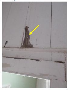
Figure 344. Cracked and flaked paint and wood bead board panels
