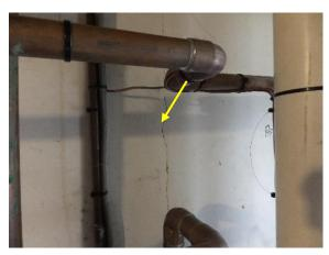
Figure 320. Parge coating cracking in mechanical area.
