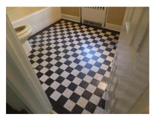
Figure 150. Checkerboard linoleum tile.
