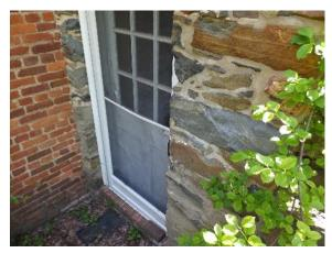
Figure 74. Cellar door and metal screen door through stone foundation.
