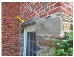
Figure 309. Wood checking at door lintel
