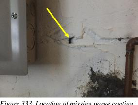
Figure 333. Location of missing parge coating from removed conduit.
