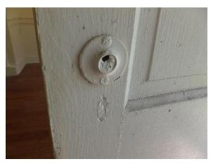
Figure 217. Remaining escutcheon from removed door knob at the south door.
