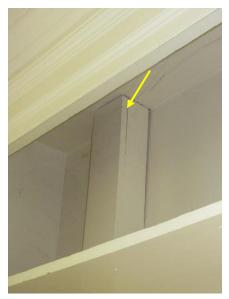
Figure 364. Splitting at vertical support member in built in cabinetry.
