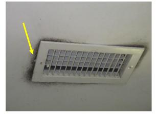
Figure 336. Potential microbial growth at ceiling vent.
