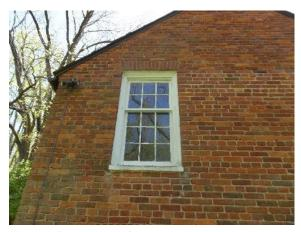
Figure 64. Typical 6/9 double hung window.
