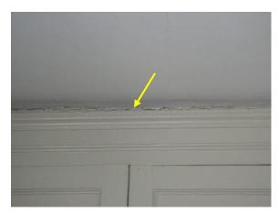
Figure 340. Separation at ceiling and cabinetry seam.
