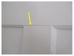
Figure 358. Separation of joinery at interior paneled door.
