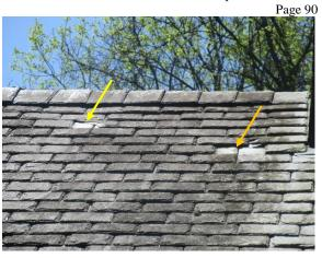
Figure 277 Broken (yellow arrow) and missing slate shingles (orange arrow).
