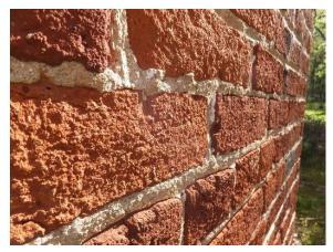
Figure 43. Rough brick and mortar surfaces at the lower brick units on the original section of the house.
