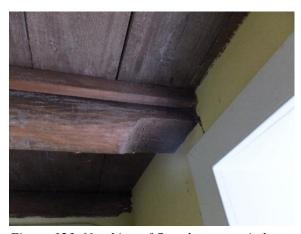
Figure 123. Notching of floor beams to timber sill.
