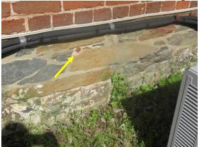
Figure 259. Varying mortar repairs at fieldstone.
