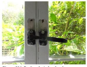
Figure 304. Replaced window hardware.
