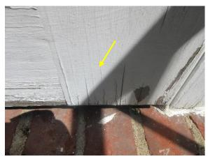
Figure 305. Cracked paint at door base.
