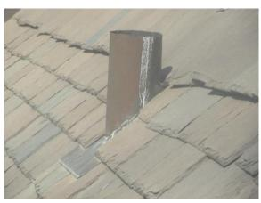
Figure 286. Pipe penetration through slate roof.
