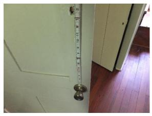
Figure 201. Contemporary pull knob added below key or hardware hole.
