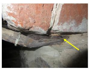
Figure 380. Corrosion product accumulation at end of curved steel fireplace lintel.
