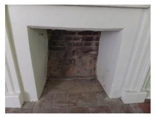
Figure 180. Parged sides of firebox.
