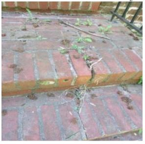
Figure 273. Cracking in mortar at brick entry steps.
