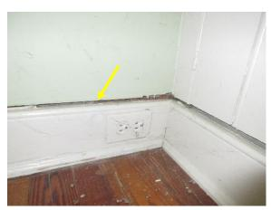
Figure 329. Gap between plaster wall finish and baseboard.
