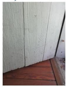
Figure 356. Weather checking at board and batten bead door base.
