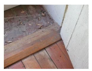
Figure 365. Weather-checking and fading varnish at door threshold.
