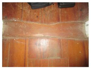
Figure 366. Well-worn threshold of east loft.
