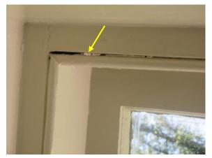
Figure 300. Separation of frame joinery (interior).
