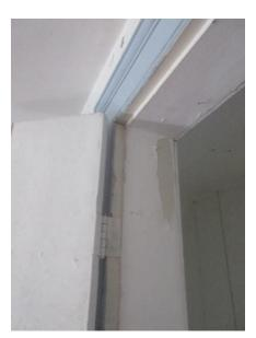
Figure 347. Flaked paint at door frame.
