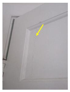
Figure 359. Crack at interior door panel.
