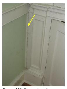
Figure 339. Separation of seams at cabinetry.
