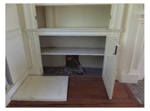
Figure 212. Lower section of cabinetry. Note trim around cabinetry to adjacent fireplace surrounds.
