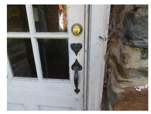
Figure 82. Typical exterior hardware at dutch doors.
