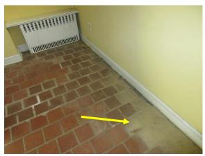
Figure 389. Staining and dirt accumulation at clay tile flooring in cellar potentially from water infiltration.
