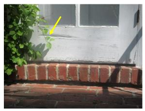
Figure 308. Crack in wood at bottom rail of storm door.
