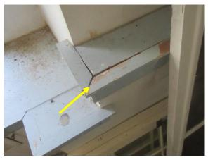
Figure 371. Separation of joinery at loft mantel.
