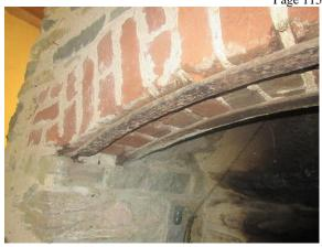
Figure 379. Surface corrosion at fireplace lintel.
