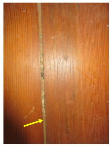
Figure 383. Wood filler at gap between floor boards at east loft.
