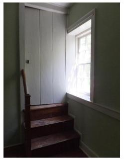
Figure 188. Board and batten bead door separating the parlor to the loft stairs.
