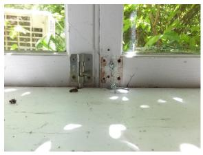
Figure 65. Contemporary barrel lock and hook added to the bottom of casement windows.
