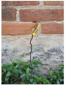
Figure 261. Crack in parge coat.
