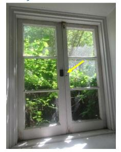
Figure 302. Missing window interior lock (interior).
