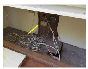
Figure 321. Cut through wall finishes for electrical at cabinetry.
