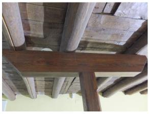
Figure 127. Retrofit T-Shaped post centered in the cellar.
