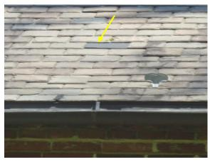
Figure 278. Metal replacement of slate shingle.
