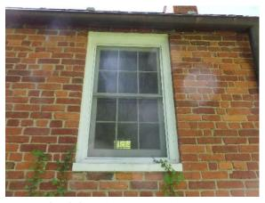
Figure 63. 6/6 double hung window at the addition with installed screen.
