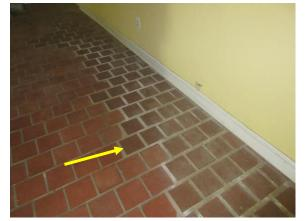
Figure 390. Replacement or staining of clay tile flooring in kitchen.
