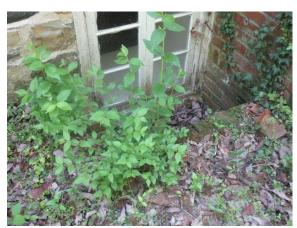
Figure 291. Foliage and debris accumulation in window well.
