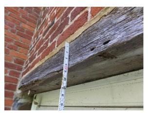
Figure 45. Large timber lintel observed at the cellar door on the west facade.
