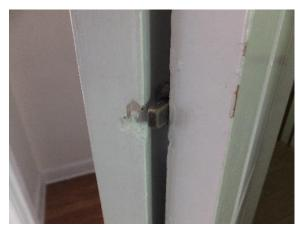
Figure 171. Damage to closet door coincidental with living space door bolt.
