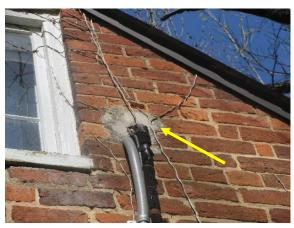
Figure 275. Conduit detailed with cementitious material at the exterior.
