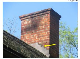
Figure 283. Mastic at copper chimney flashing.
