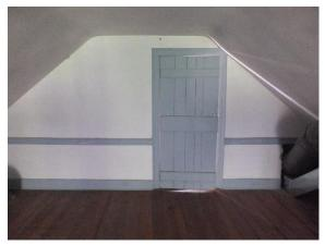
Figure 250. View of the loft east board and batten bead door as view from inside the room.
