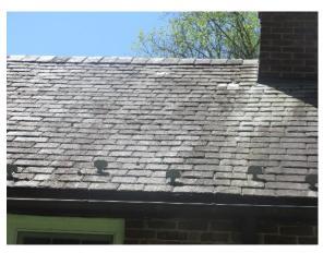
Figure 52. Copper gutters and snow guards.
