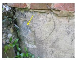
Figure 262. Spall in parge coat.
