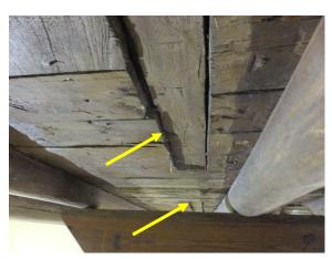
Figure 129. Interruptions of subfloor that correspond with interior wall between the hall and parlor.
