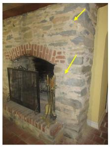
Figure 355. View of mortar campaigns at cellar fireplace.
