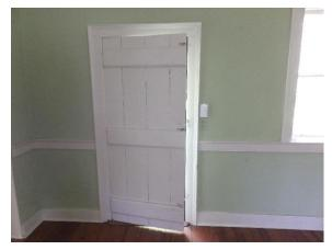
Figure 72. Interior view of the same board and batten bead door in the Parlor.
