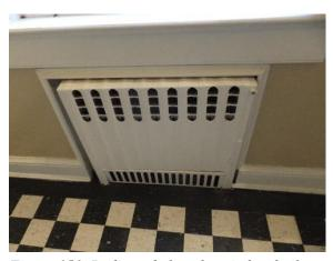
Figure 151. Radiator below the window built into the wall. This configuration is typical in the 1941 addition at this level.
