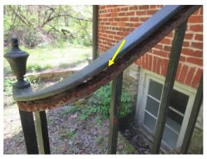
Figure 312. Corrosion and material loss at hand rail.
