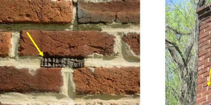
Figure 268. Wood element, possibly a shim, in a mortar joint at the original section of the home.
