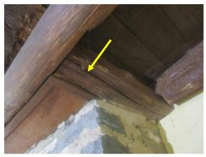
Figure 376. Wood splintering/splitting at original beams framing the cellar fireplace.
