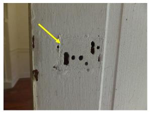
Figure 218. Holes and ghosting from a removed surface mounted lock, such as a rim lock, at the south door.
