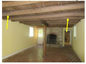
Figure 373. Overall view of wood joists and various splitting of 3/4 round floor beams.
