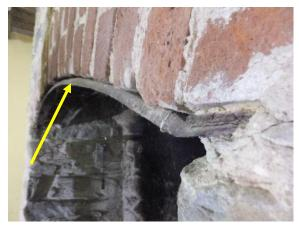
Figure 134. Iron chimney bars.
