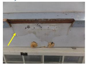
Figure 239. Evidence of a removed wall-mounted sink.
