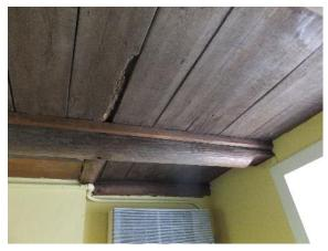
Figure 128. Retrofit of wood member between beam and subfloor.
