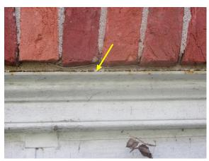
Figure 296. Surface corrosion at window lintel.
