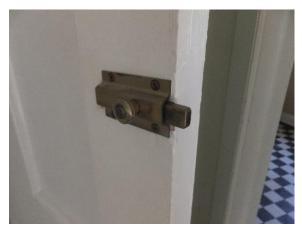
Figure 159. Bolt latch hardware on interior side of door.
