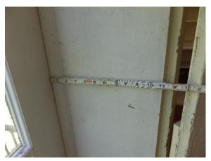
Figure 216. Door casing that is 12 inches wide to accommodate the thickness of the brick wall.
