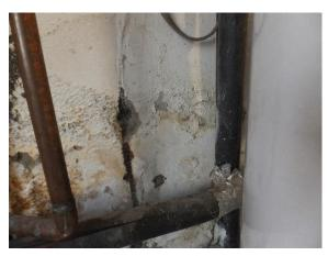
Figure 334. Water staining, blistering and cracking of parge coating.
