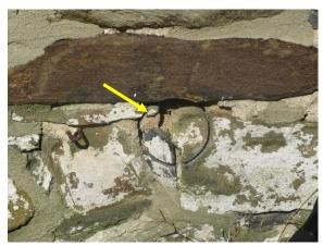
Figure 263. Abandoned attempt at a core drill for a penetration.
