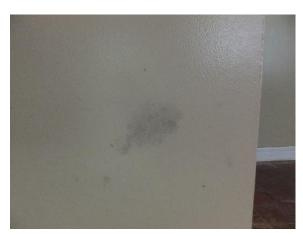
Figure 342. Staining at wall paint.
