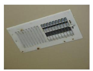
Figure 393. Surface corrosion of vent and fasteners at bathroom.
