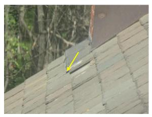
Figure 285. Lifted chimney flashing edge and adjacent slate shingle.
