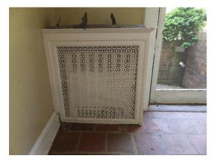
Figure 114. Radiator within a cabinet with a stamped metal grille.
