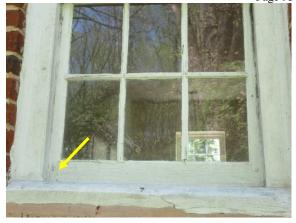
Figure 293. Separation of frame joinery.
