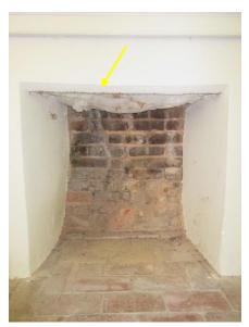
Figure 351. Insulation installed at the throat of parlor fireplace.
