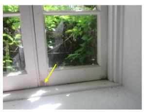
Figure 301. Peeled paint at window (interior).
