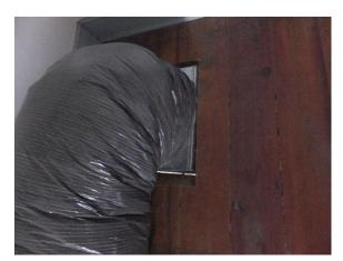
Figure 255. Ductwork penetration through the wood floor was observed in both loft rooms.
