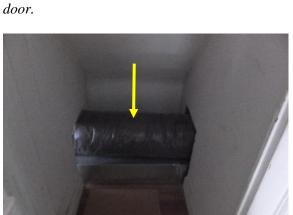
Figure 235. Ductwork running through the closet walls.
