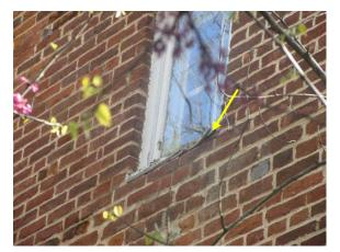
Figure 298. Deteriorated window sill.
