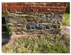
Figure 44. Stone foundation exposed at the original section of the house.
