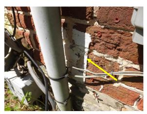
Figure 40. Remnant white coating observed at the east facade behind conduit.
