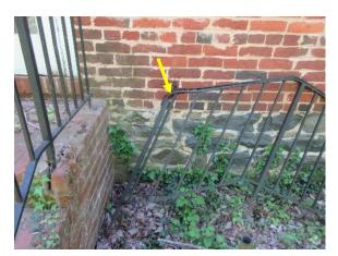
Figure 313. Detached metal railing.
