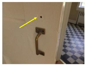
Figure 160. Typical pull handle on interior side of door with hole from other removed element above.
