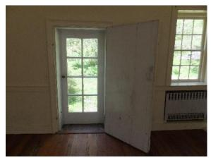
Figure 73. View of the exterior of the board and batten bead door in the Hall with glass lite storm door.
