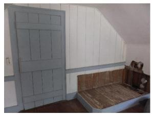
Figure 248. Paneled wood bead board at the east wall.
