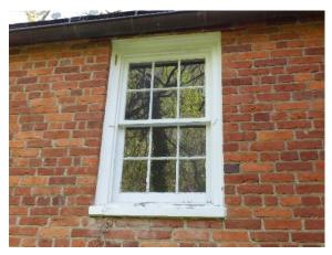
Figure 62. 6/6 double hung window at the addition. Note pivot hardware.
