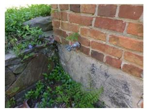
Figure 49. Exposed parged CMU foundation at the west facade.
