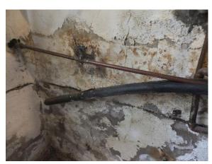
Figure 331. Flaked coating and staining at parge coating at mechanical area.
