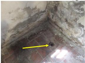
Figure 391. Abandoned penetration at clay tile flooring in utility room.
