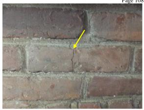
Figure 349. Vertical cracking at brick and mortar at kitchen fireplace.
