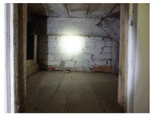
Figure 195. View into area below the stairs. Note white coating on south wall brick.
