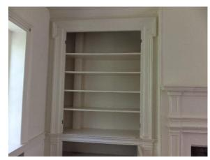
Figure 211. Built-in cabinetry to the north of the fireplace. Note missing upper doors.
