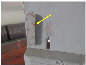
Figure 363. Surface corrosion at original bar strap at board and batten bead door.
