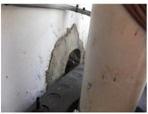
Figure 326. Cementitious material at cut in parge coating for abandoned penetration.
