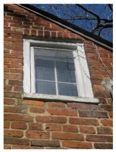
Figure 290. Overall view of exterior storm window at loft window.
