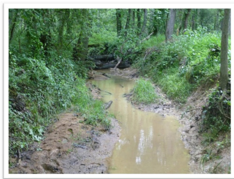
Sedimentation downstream of log structure installed in November of 2012 at Huntley Meadows Park. Photo taken June 2013.
