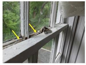
Figure 45. Muntin deterioration at upper sash meeting rail.
