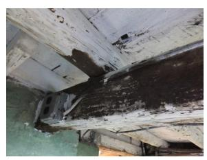
Figure 78. Dark stain on beam in cellar, adjacent to chimney. Note white coating on original 3/4 round beams and underside of first floor.
