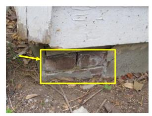
Figure 27. Spall in parge coat allowing the brick to become exposed.
