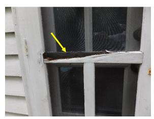
Figure 31. Missing section of wood at the horizontal member of an east screen door.
