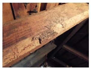
Figure 79. Damaged edge of rafter potentially from pest activity.
