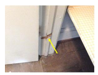
Figure 98. Gouge in door frame at door D103.
