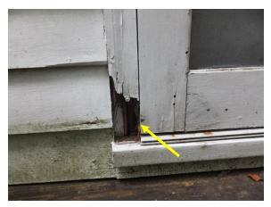
Figure 32. Missing section of wood at the base of an east screen door.
