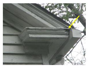
Figure 12. Deteriorated wood at cornice element on northwest corner behind gutter.
