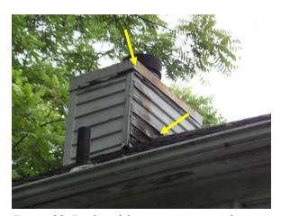
Figure 28. Dark and ferrous staining at the chimney.
