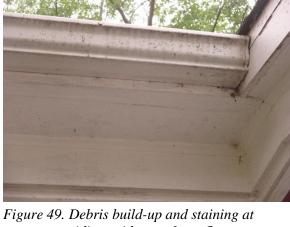
gutters providing evidence of overflow.
