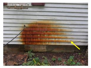
Figure 18. Ferrous staining on east facade adjacent to water spigot.
