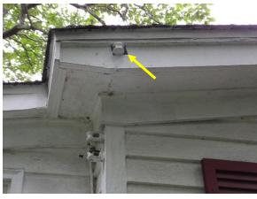
Figure 25. Rough opening through the cornice for the utility line anchor.
