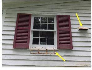
Figure 19. Corrosion on metal elements attached to facade due to deteriorated coatings.
