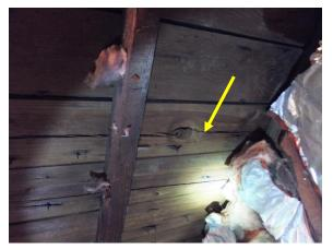
Figure 83. Cracked decking timber in attic.
