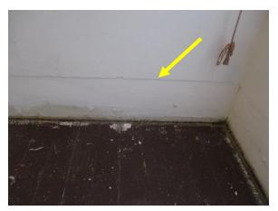
Figure 61. Typical condition in rooms that are missing baseboards: paint build-up line across wall and scraped paint at bottom of baseboard.
