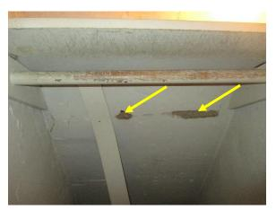
Figure 67. Missing plaster below the stairs revealing the wood lathe.
