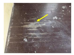
Figure 93. Paint scraped from wood floor.
