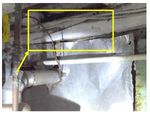
Figure 77. Full-depth split through timber sill in cellar.
