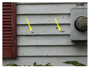
Figure 17. Typical paint deterioration on wood siding with some areas of wood exposed.
