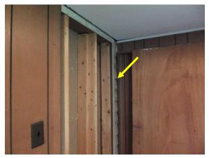
Figure 73. Panel able to be easily removed reveals the original exterior door location when room 103 was an open porch. Note exterior wood siding still in place.
