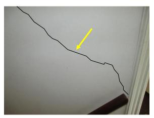
Figure 64. Diagonal cracking in stairwell. Crack traced for clarity.
