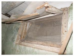
Figure 48. Window in basement that is not visible from exterior and may be infilled. Deteriorated wood can be seen around the frame.
