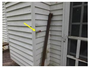
Figure 15. Area of deteriorated wood siding at the east chimney.
