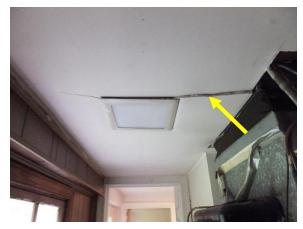
Figure 58. Crack and vertical displacement in ceiling at lighting fixture in room 104 (enclosed north porch).
