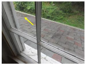
Figure 51. Vegetation growing on the roof at the second roof on the north.
