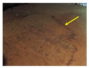
Figure 85. Stain from previous water infiltration on west attic floor.
