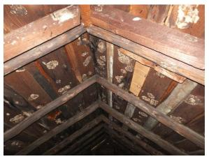
Figure 87. Historic peeled log rafters toe-nailed without a ridge beam or board in attic.
