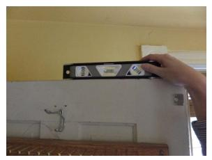
Figure 103. Door in room 200 on second floor is not plumb.
