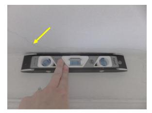
Figure 70. Sloped ceiling in second floor hallway, note cracking in finishes.
