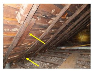
Figure 86. Peeled log rafters in attic with additional milled lumber for decking.
