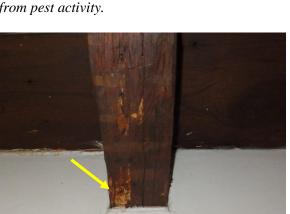
Figure 81. Deteriorated wood in room 101, potentially due to pest damage.
