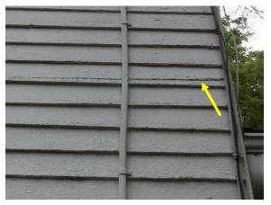
Figure 22. Split in wood originating from southwest corner.
