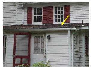
Figure 52. Soiling of asphalt shingles at the secondary roof on the south.
