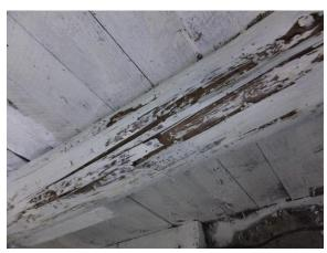
Figure 74. Soft and splintered 3/4 round beams in cellar.
