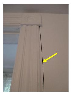
Figure 57. Crack in plaster around door frame on second floor. Crack traced for clarity.
