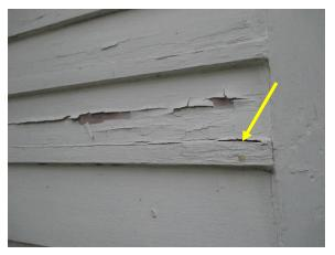
Figure 21. Split in wood originating from edge of wood board above fastener.
