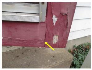
Figure 30. Typical separation of joinery at doors.
