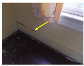
Figure 62. Horizontal cracking at location of previous baseboard in room 200.
