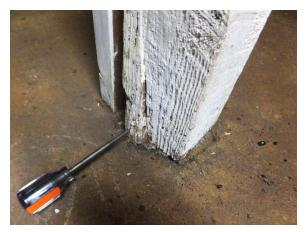
Figure 75. Soft and split wood at base of solid sawn column in cellar. Retrofit manufactured wood piece has been installed adjacent to the original column.
