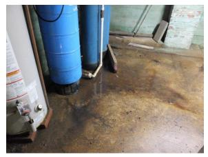
Figure 90. Water pooling on concrete floor in cellar.
