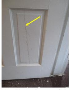
Figure 96. Crack through panel of a historic interior door.
