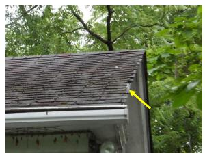
Figure 53. Missing shingles at the edge of the south gable.
