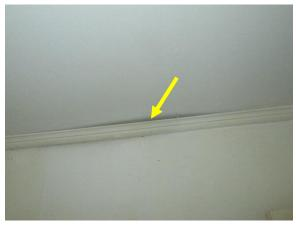
Figure 63. Separation of crown molding from ceiling and wall.
