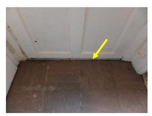
Figure 102. Water staining at base of exterior door D110.
