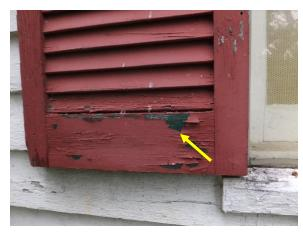
Figure 41. Typical deterioration of paint on window shutters revealing previous green paint.
