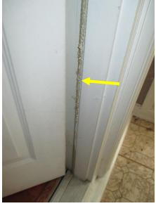
Figure 101. Deterioration of seal at door D106.
