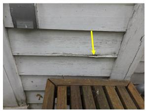
Figure 13. Deteriorated wood siding on east facade, adjacent to chimney.
