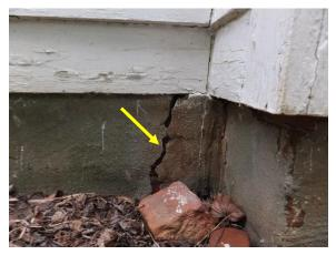
Figure 26. Crack and delamination in parge coat that covers brick foundations.
