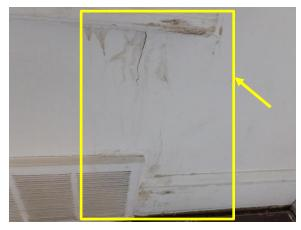
Figure 66. Evidence of water infiltration on interior finishes with related cracking on the second floor.
