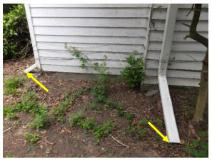
Figure 50. Downspouts terminate near the foundation without any splash pads.
