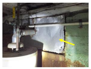
Figure 91. Unsealed ventilation window opening in cellar below-grade wall.
