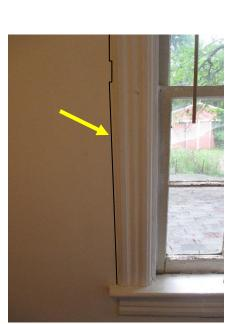
Figure 59. Crack in plaster wall around window frame on second floor. Crack traced for clarity.
