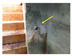
Figure 88. Spall at pipe penetration at concrete in cellar.
