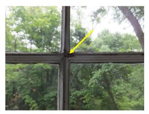
Figure 44. Typical deterioration of muntins at interior.
