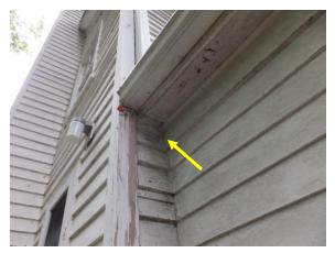
Figure 14. Deteriorated wood soffit and siding beneath gutter at south east corner.
