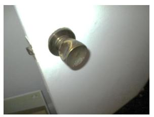
Figure 99. Crushed door knob at door D115.
