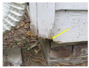
Figure 11. Deteriorated wood at trim element on corner. Note exposed brick at foundation where parge coat and brick mortar are no longer intact.
