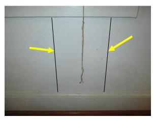
Figure 60. Cracks in plaster beneath window sill. Cracks traced for clarity.
