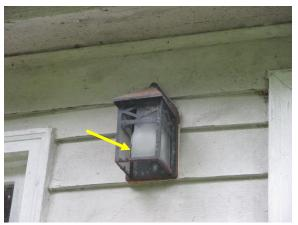
Figure 56. Lighting fixture on north facade with cracked glass at front.
