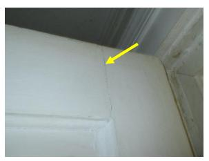
Figure 95. Typical separation of joinery at historic interior doors.
