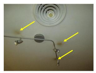
Figure 68. Burn marks on ceiling at room 100 above the light fixture.
