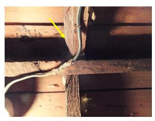
Figure 82. Rotated rafter in west attic.
