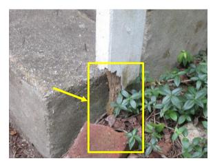
Figure 35. Missing section of wood at the southeast exterior door handrail post.
