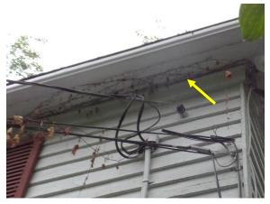
Figure 10. Vegetation underneath eave and along the power lines at the west facade.
