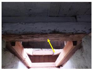
Figure 76. Deteriorated wood at underside of timber sill at hatch to cellar.
