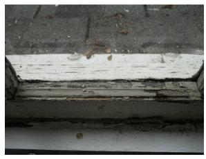
Figure 43. Typical paint and glazing putty deterioration at windows.
