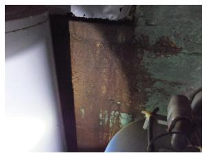
Figure 89. Rust staining on concrete wall in cellar.
