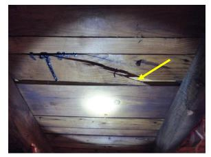
Figure 84. Split decking timber in attic.
