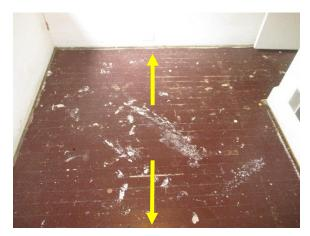
Figure 94. Sloped floor in room 202.
