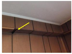
Figure 72. Delamination of wood panel at the soffit in room 103.
