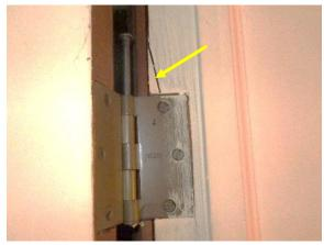
Figure 97. Crack at hinges of door D113. Hinges also appear to be misaligned with the pin not fully engaged.
