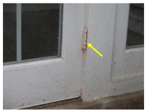
Figure 34. Corroded hinges at southwest french doors, typical condition for exterior doors on the home.
