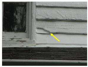
Figure 23. Missing section of wood siding with metal flashing below on north facade.
