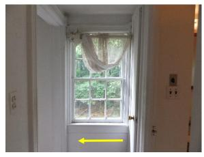
Figure 37. Window 204 sloped to the west.
