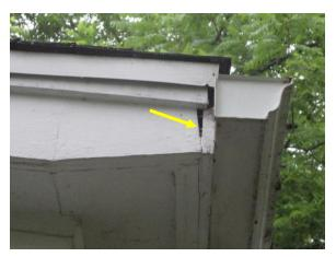
Figure 24. Separation of wood fascia board adjacent to the gutter.
