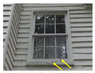
Figure 40. Typical flaked paint on window elements and frame.
