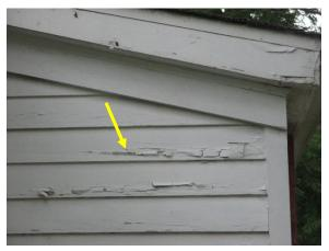
Figure 16. Typical paint deterioration on wood siding.
