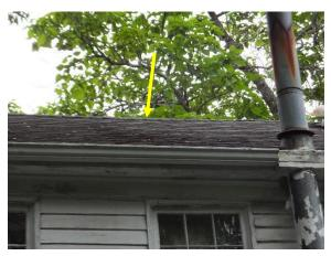
Figure 54. Low spot on main gabled roof above the Period I section of the home.
