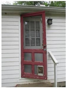
Figure 29. Typical paint deterioration of exterior doors.
