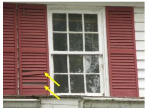
Figure 42. Broken and missing slat on shutter at south facade.
