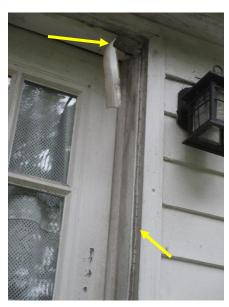
Figure 33. Deteriorated weather seal for screen door on southeast exterior door.
