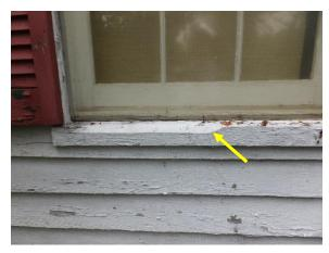
Figure 46. Area of missing wood at a first floor window sill on west facade.
