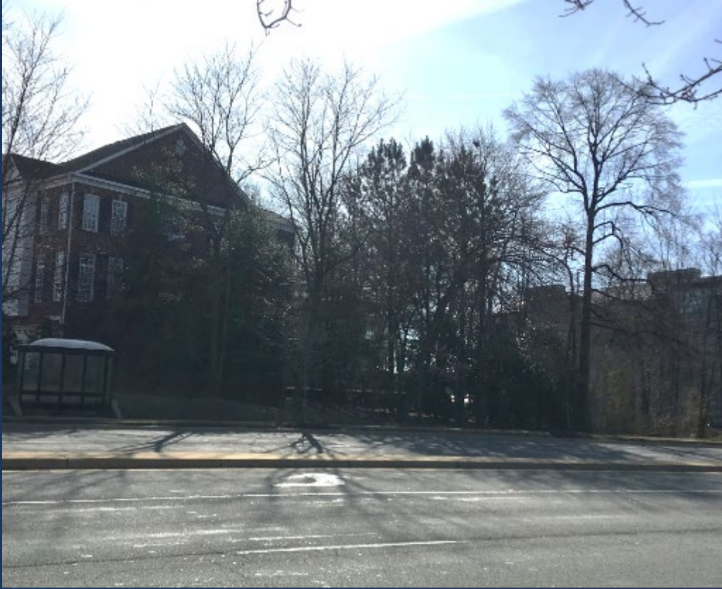
Fairfax Gateway development, view across Route 123 from subject area
